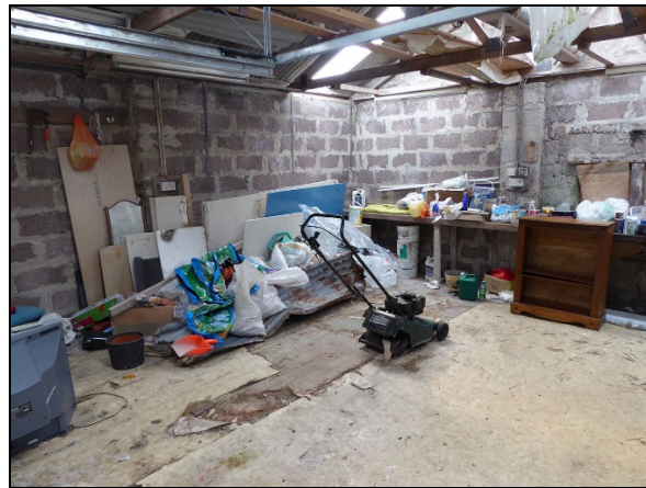
Interior of Garage
