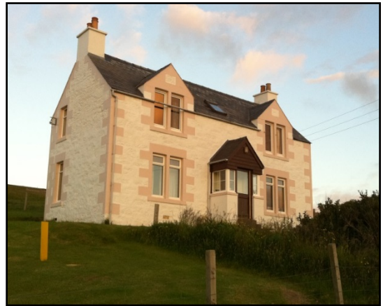
The outside was repainted in September 2015
